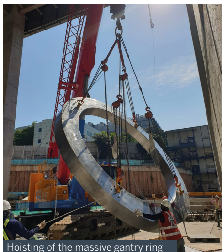
Installation of the Proton Gantry
