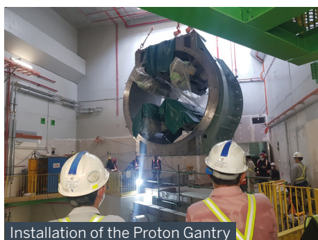
Installation of the Proton Gantry
